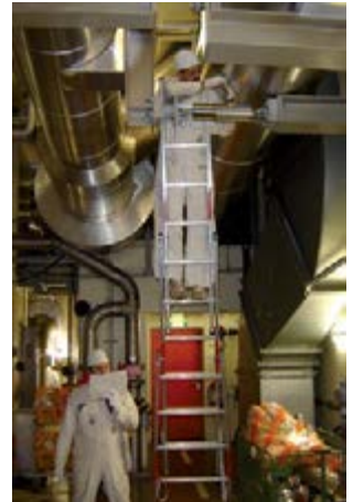
Visual inspection of snubbers
