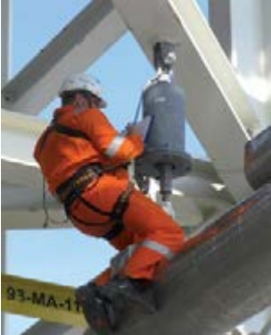
Controlling a pipe support
