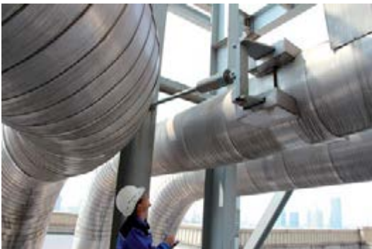
Inspection of supports at the plant
